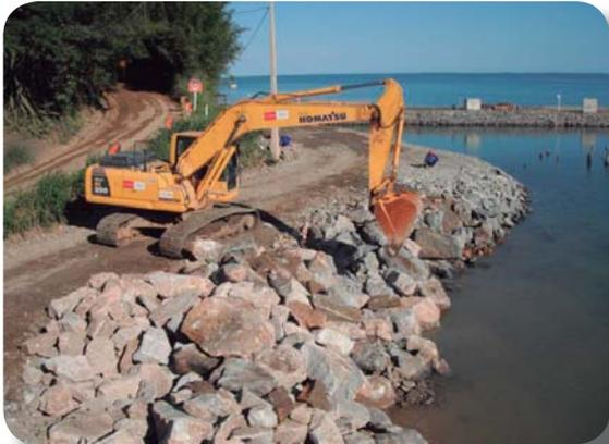
Figura 4 – Enrocamento<sup>(2)</sup> (PROSUB/EBN)
