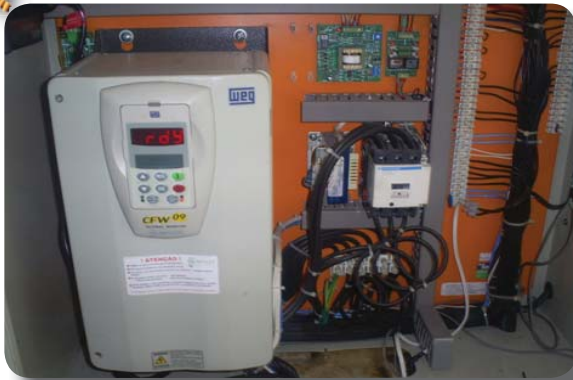
Figura 6 – Painel de controle microprocessado (FERREIRA, 2010)
